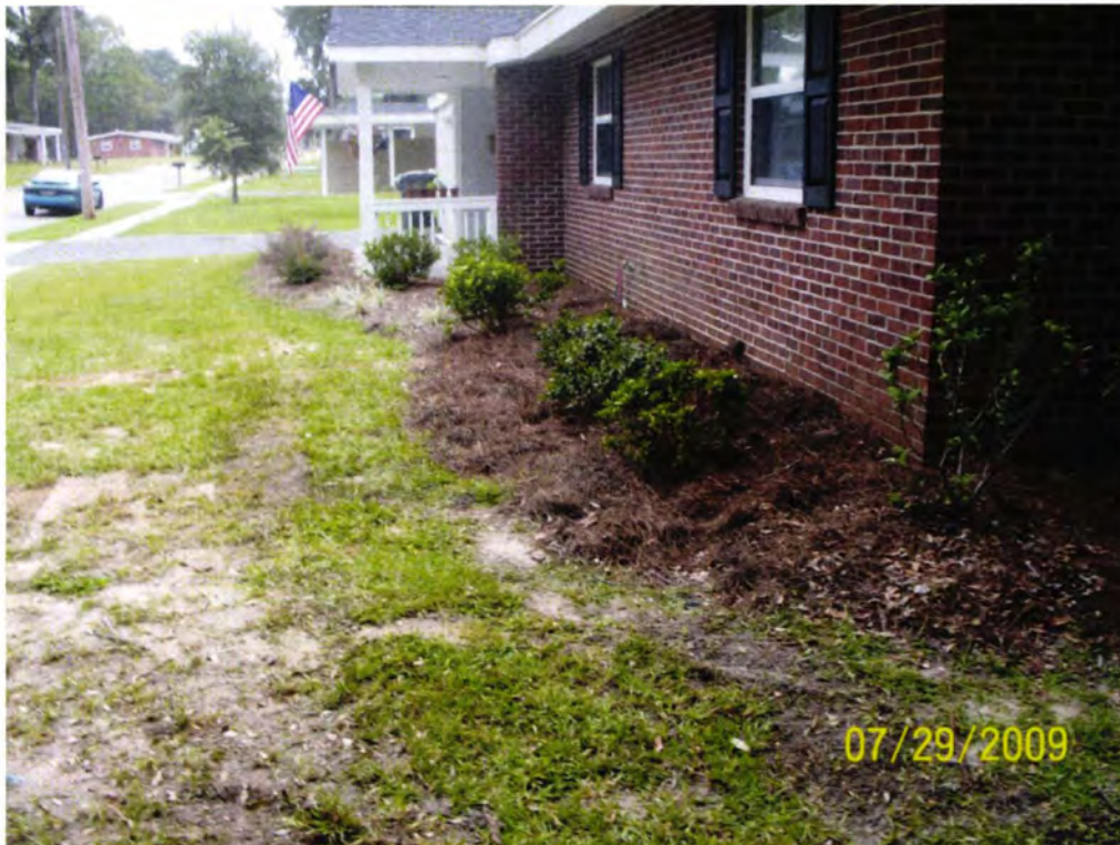
Picture 2: Site after completion of work.
