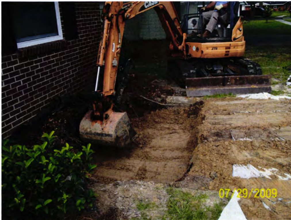
Picture 1: UST 1406Eagle during backfill.
